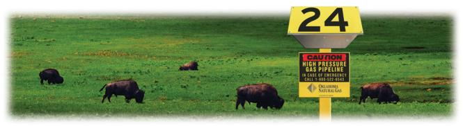
A pipeline right of way is a strip of land over and around buried pipelines that allows them to be permanently located on public and/or private land to provide natural gas service. Rights of way should be kept clear of obstructions to enable Oklahoma Natural Gas employees to safely operate, patrol, inspect, maintain and repair natural gas pipelines.
